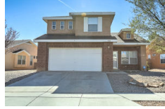
7508 Breckenridge Road NW Albuquerque NM
