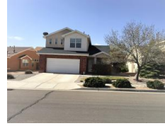
7516 Breckenridge Road NW Albuquerque NM
