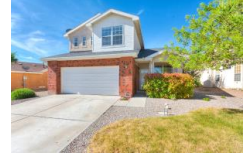
7516 Breckenridge Road NW Albuquerque NM
